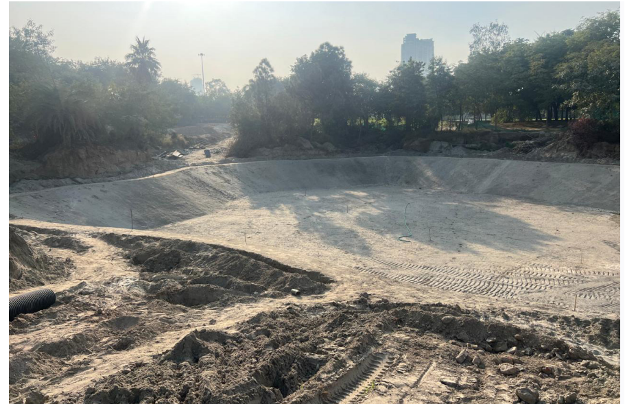
Figure 10: Excavation and shaping of one of the new irrigation lakes (Source: Golf Design India)
