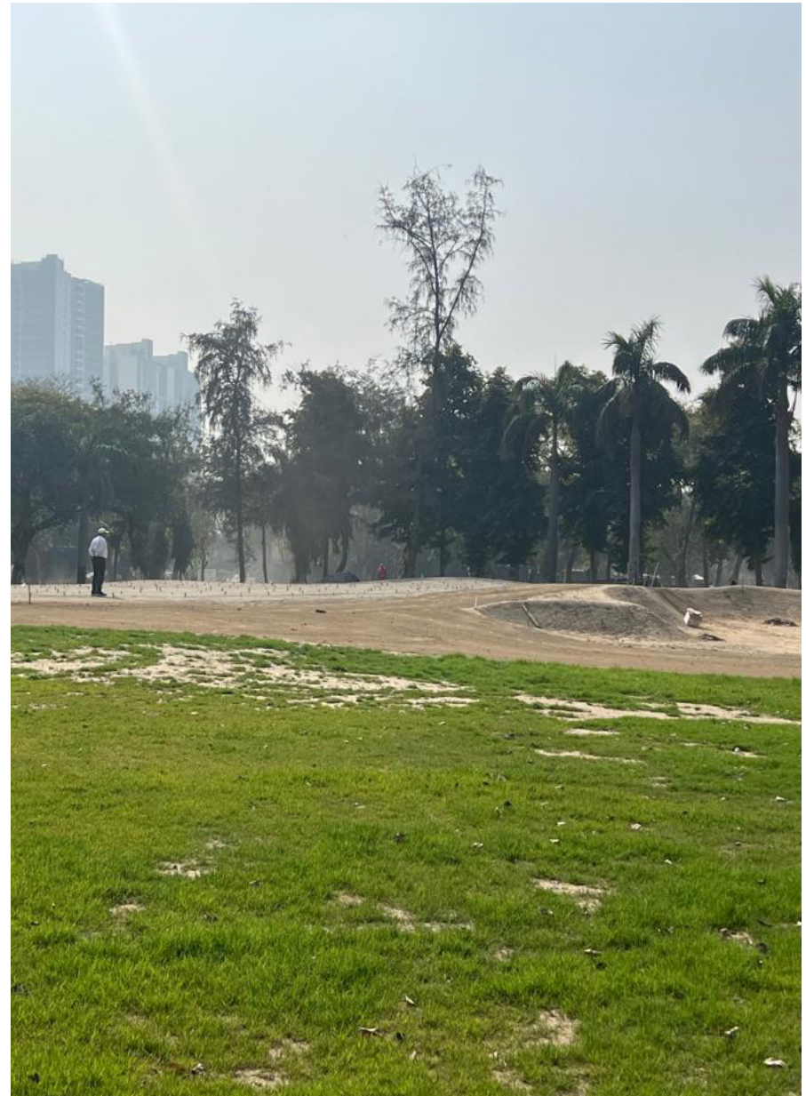
Figure 15: Green and bunker shaping on site (Source Golf Design India)
