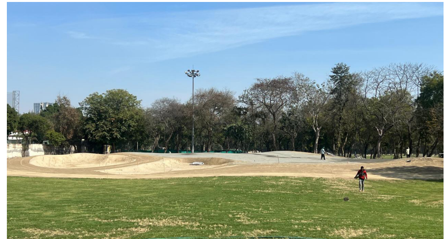
Figure 13 - Construction of new greens complexes (Source Golf Design India)
