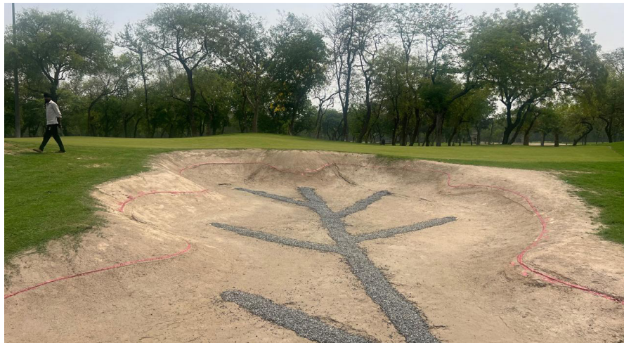
Figure 12 - New drainage being installed in a bunker (Source Golf Design India)
