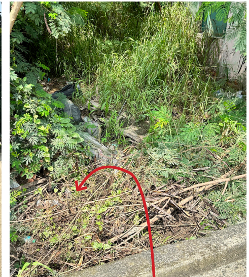
Drainage ditch that has become full of vegetation and debris, blocking the flow of run off water significantly.
